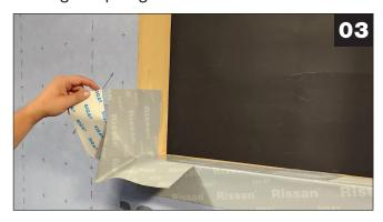
Remove remaining backing paper, and pull corner gusset onto the face of the sheathing
