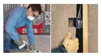
Roxul cuts quickly and accurately with a serrated knife, such as a bread knife, so you can easily achieve optimal fit around pipes, electrical boxes, wiring, ductwork, and between studs and joists that are less than a standard width.
