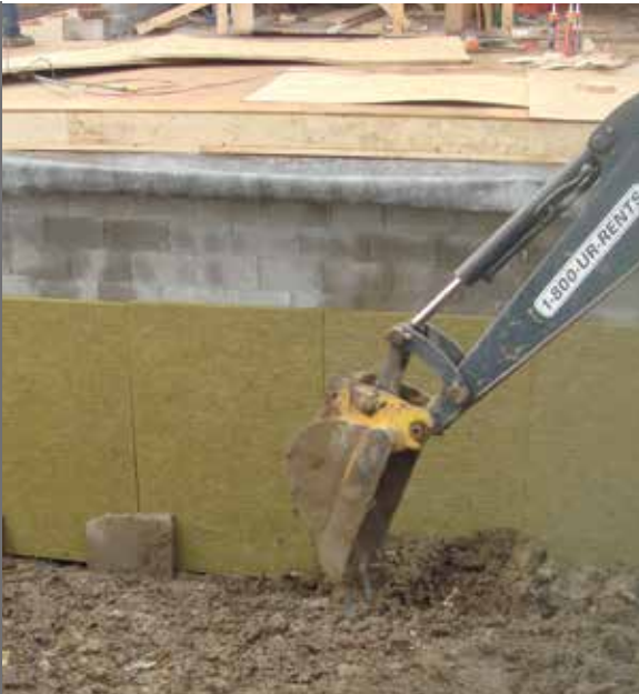
The superior strength of DRAINBOARD also means it is very resistant to damage during installation and backfilling operations.
