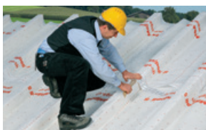
Mounting vapour control layer for roof renovation from the outside
