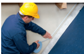
Joining roof underlay membrane to solid wall construction
