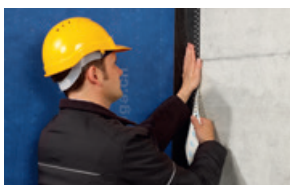
Joining facade membrane to solid wall construction
