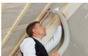
Mounting vapour control layer for injection insulation
