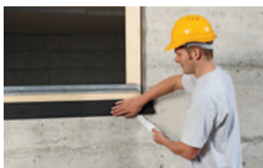
Joining window to solid wall construction
