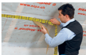
Vapour control layer overlaps
