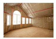
ROXUL COMFORTBATT\* is a semi-rigid batt insulation designed specifically for exterior wood and steel stud applications in residential and commercial construction. Made from natural stone and recycled slag, ROXUL stone wool is a high density insulation that will fit snugly into wall cavities and will not slump over time. It also adds superior acoustical performance to wall assemblies and floors and can be used in acoustic applications required by building code.
