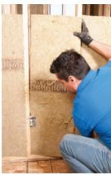
ROXUL® cuts quickly and accurately with a serrated knife, such as a bread knife, so you can easily achieve optimal fit around pipes, electrical boxes, wiring, ductwork, and between studs and joists that are less than a standard width.
