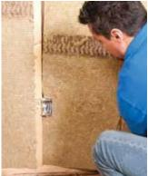
ROXUL COMFORTBATT® higher density batts make it simple for precise cutting to ensure a fit without gaps and voids.
