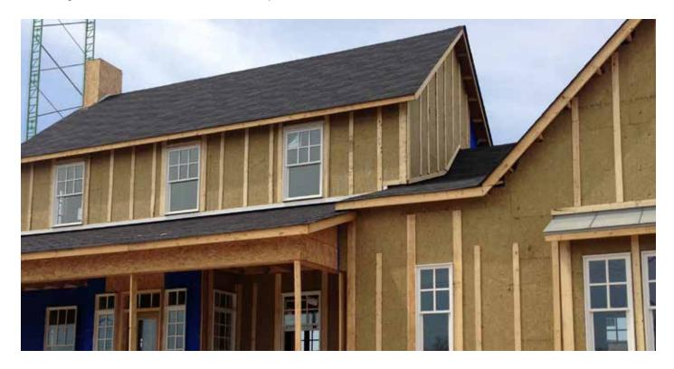
be. Wherever possible, the exterior insulation ratio should be maximized. This can mean the use of thicker exterior insulation over an insulated 2x4 wall instead of
