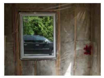
Typical polyethylene plastic sheet (Class I vapour retarder) installed on the interior of a 2x6 insulated wall in Canada
