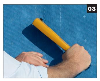
Minimum overlap for vertical and horizontal seams is 4"
