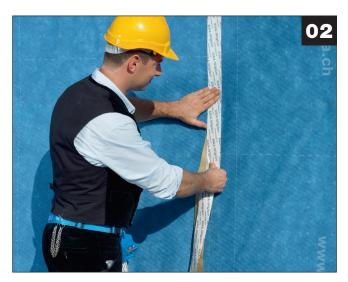
Apply it without tension and creases and press on firmly with hand pressure
