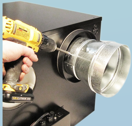
2. Add 8" - 6" Reducer & Secure with Tek Screws
