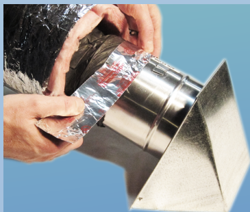
3. Tape Inner Duct
