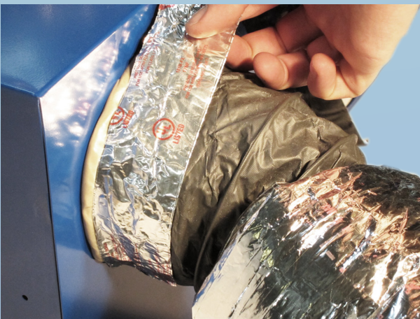
3. Tape Inner Duct to Collar
