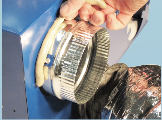
2. Use Mastic Putty to Seal Collar to Ventilation Unit
