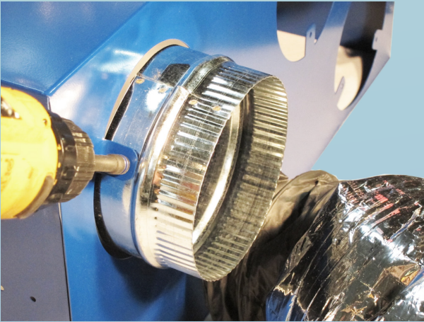
1. Attach Starter Collar to Ventilation Unit by Bending Tabs & Secure With Self Drilling Tek Screws
