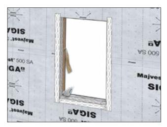
Remove second backing strip and apply tape on jambs while firmly pressing on with a roller or squeegee.
