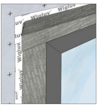
Remove one backing paper and apply the tape along the top of the window while applying firm pressure.
