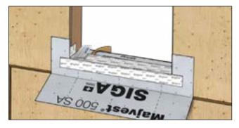
Remove second backing strip and apply tape on sill while firmly pressing on with a roller or squeegee.
