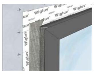
Cut Fentrim 230 grey about 4" wider than the width of the prepared rough opening so both ends are overlapping the tape on the jamb.
