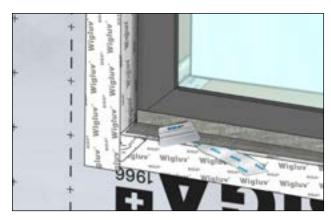
Press on firmly while removing the second backing strip.
