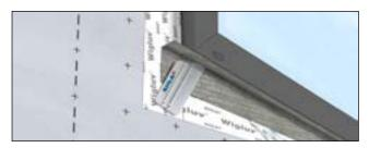
Remove backing paper and press on firmly using a roller or squeegee.
