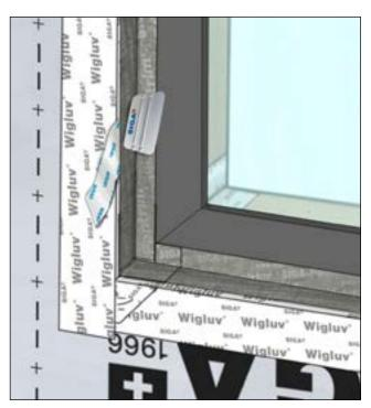
Remove backing strip and press on tape firmly using a roller or squeegee — repeat on both sides.
