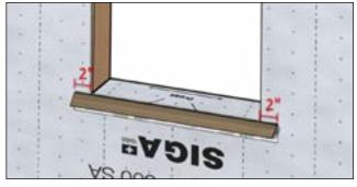
Cut Wigluv 4" wider than the sill so it will extend 2" past each end of the rough opening.
