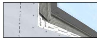
Cut Fentrim 230 grey about 2" wider than the vertical portion of the rough opening. Apply narrow side of the tape along the window while applying firm pressure.
