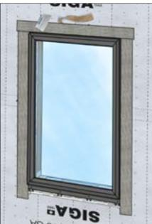
Remove second backing strip while applying firm pressure using a roller or squeegee.
