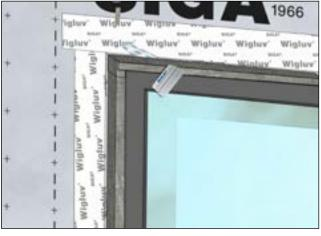
Remove backing paper and work tape onto the pre-flashed top, do not install tape with tension, press on firmly.
