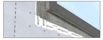
Fold both ends up and apply firm pressure. Repeat on both sides.
