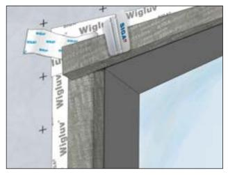
Remove larger backing paper and press on firmly using a roller or squeegee.
