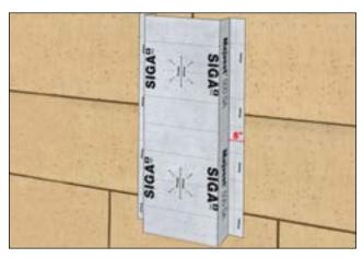
Install Majvest 500 SA while leaving at least 8" overlap on all four sides. Press on using a roller or squeegee.
