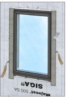
Remove second backing strip and apply firm pressure using a roller or squeegee.
