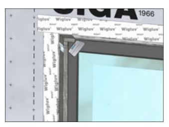
Apply 3D corner boot in top corner while applying firm pressure — repeat on both sides.
