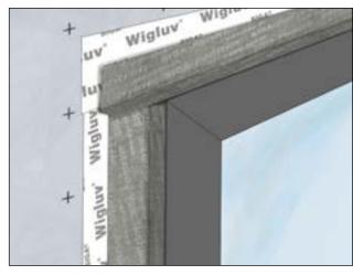
Apply narrow side of the tape along the top of the window while applying firm pressure.
