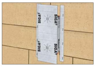
Flap 4 middle sections inside on the extension buck and press on firmly.
