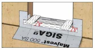
Create two gussets with Wigluv 100 by cutting a piece of tape that's the full depth of the rough opening plus 3".
