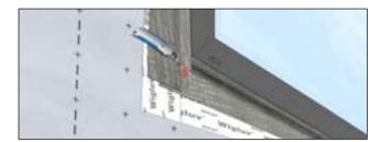
Remove backing paper and press on firmly using a roller or squeegee. Make 45° cuts at each end, from the inside corner outwards, make sure to not cut the tape too deep to avoid pinholes.
