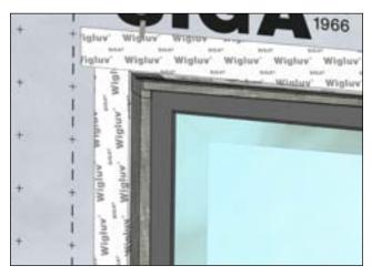
Cut a strip of Fentrim 230 grey as long as the horizontal portion of the rough opening. Apply pre-folded tape section along the horizontal portion of the frame.
