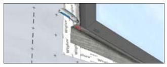
Make 45° cuts at each end, from the inside corner outwards, make sure to not cut the tape too deep to avoid pinholes.
