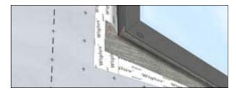
Fold both ends up and apply firm pressure.
