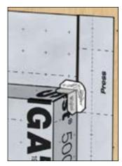
Use 4" long tape strip and apply into corner while using the stretch of Wigluv.
