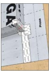
Fold remaining tape section onto the bottom of the extension buck. Apply pressure.
