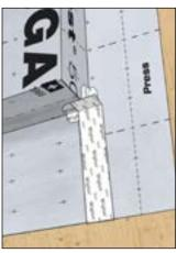
Tape membrane with Wigluv 100 and overlap
