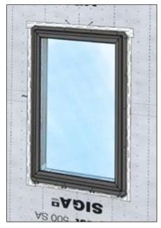
Install flanged window on flashed rough opening as per manufacturer's recommendation. For flanged windows the sill is rarely taped, check with the window manufacturer before tape installation.
