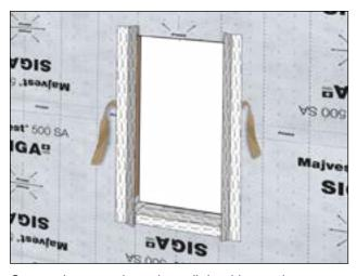
Crease the tape along the split backing and remove one backing strip.
