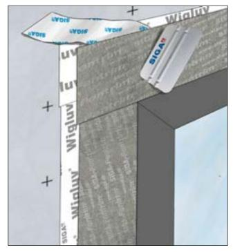
Remove second backing paper and press on firmly using a roller or squeegee.
