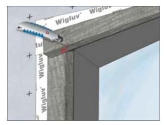
Make 45° cuts at each end, from the inside corner outward, make sure to not cut tape too deep to avoid pinholes.
