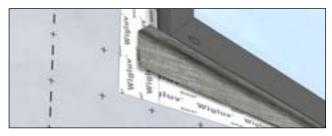
Cut Fentrim 230 grey about 2" wider than the width of the prepared rough opening. Apply narrow side of the tape along underside of the window while applying firm pressure.
